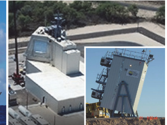
Aegis Ashore and Vertical Launch System
