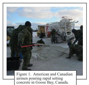
This event demonstrated the ability to rapidly repair an airfield as well as the durability of repairs through simulated C-17 airlifter traffic. This test illustrates the value of ITEP in sustaining operational capability under realistic, adverse conditions (Figure 2).
