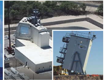
Aegis Ashore and Vertical Launch System
